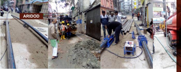
Dhaka Water Supply and Sanitation Development Project (DMA 310 & 309) Ludwig PFEIFFER HDPE Pipe laying by HDD & OC Method
