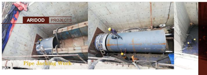
Pipe Jacking Work of 33KV XLPE Power Cable & Water Pipe Through 2050mm Outer Dia MS Pipe beneth Dhaka Chittagong **Double Track Rail Line**
